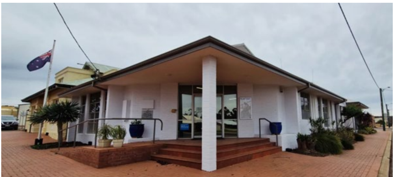
Shire Admin Office External Painting
