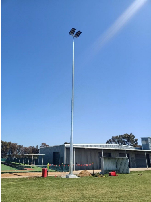
Oval Lighting Upgrades Kukerin & Dumbleyung
